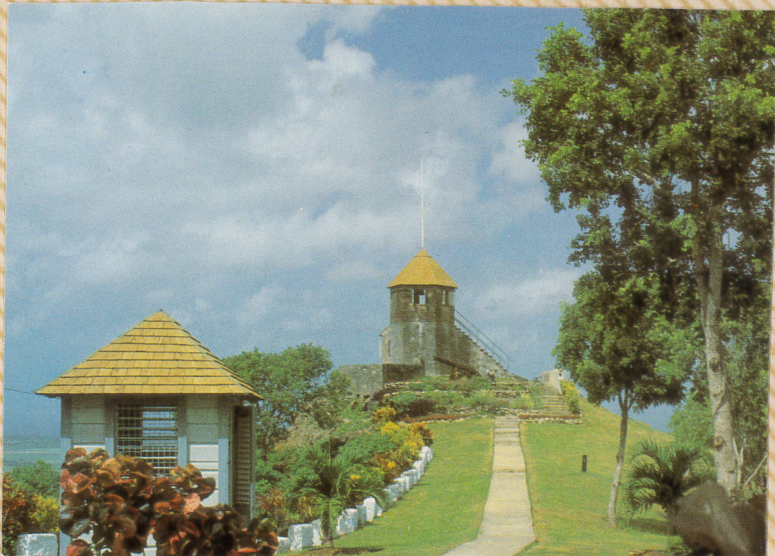
Gunhill Signal Station, St. George, Barbados, West Indies. Restored and maintained by the Barbados National Trust.
